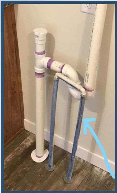
Water Softner Prep w/ Drain & Recept
