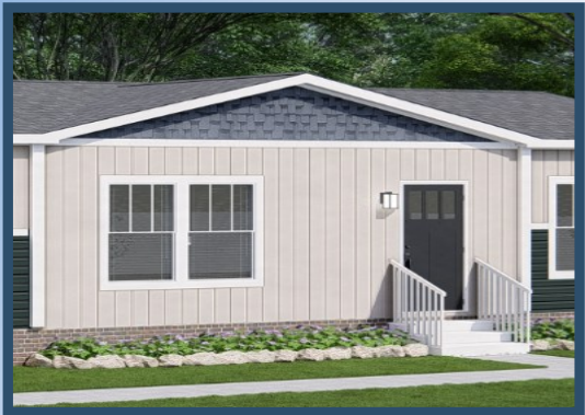
Shake Siding on Dormer Above
