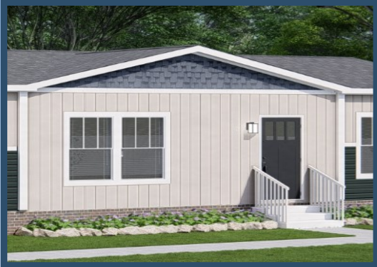
Shake Siding on Dormer Above
