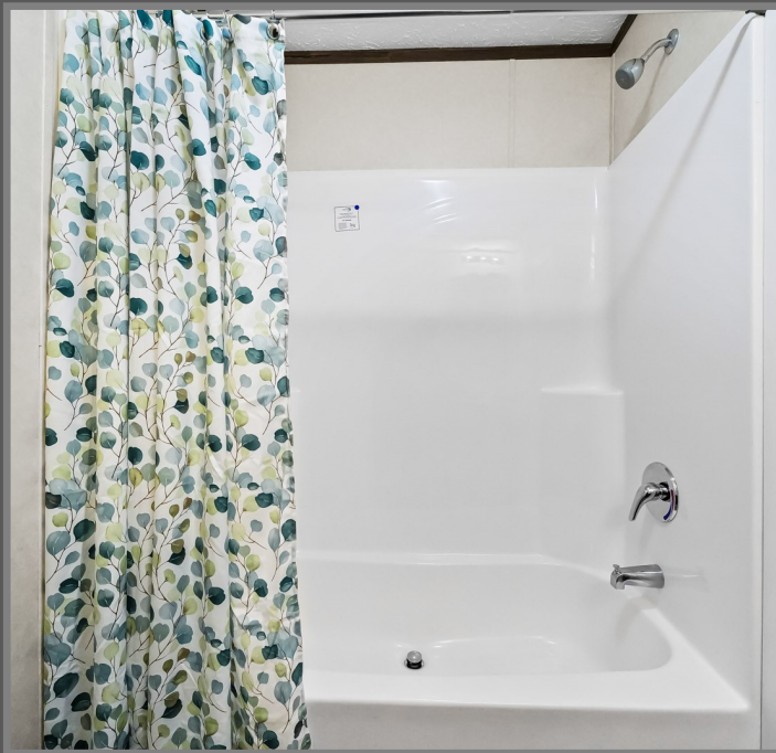
60" Fiberglass TUB /SHOWER Bath 1 & Bath 2 No Drape Available
