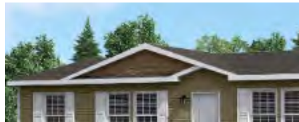
Shake Siding on Dormer above Continuous Eave
