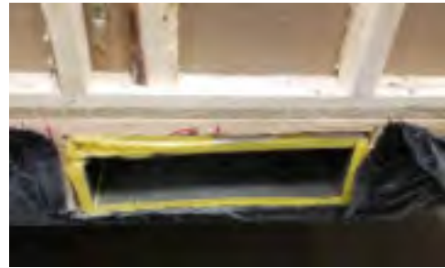
Fiberglass Heat Ducts w/ In Floor Cross over Heat Ducts - HUD ONLY
